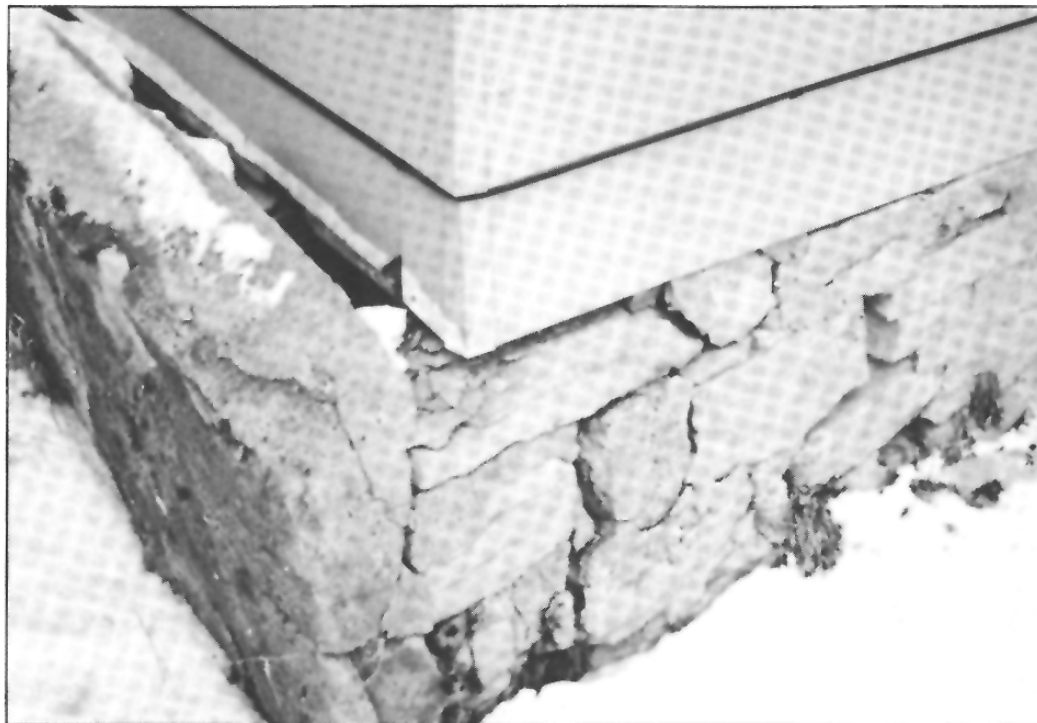
Figure 304.5 MAJOR DAMAGE TO A FOUNDATION WALL This foundation is crumbling. Failure to repair it will eventually lead to its collapse.
